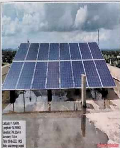
Solar System installed - Main Building 10KW
