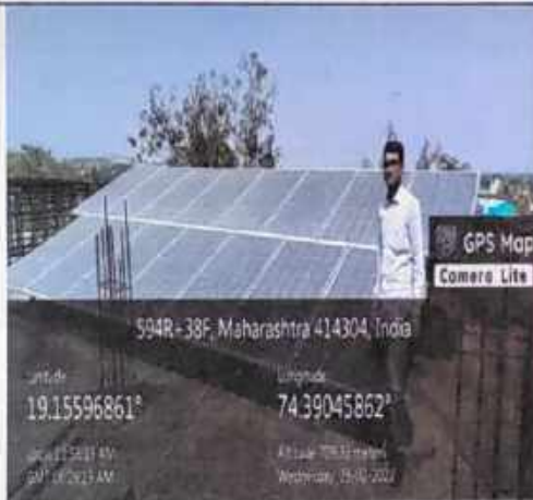
Solar project-Ladies Hostel 5KW
