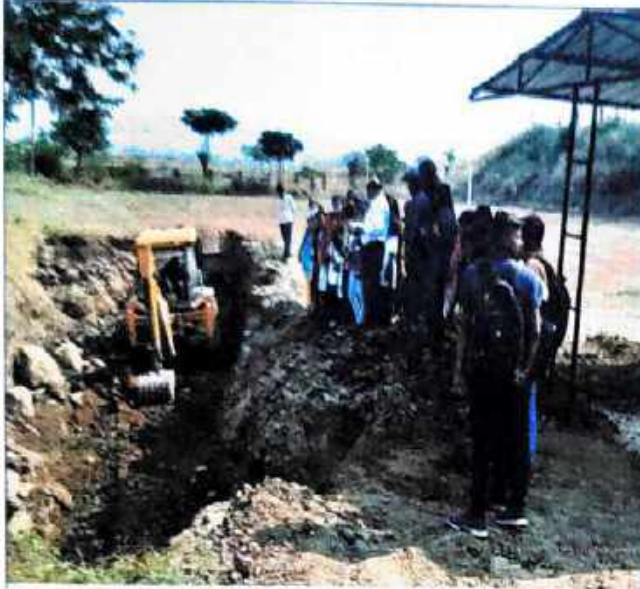
Principal giving information to the students while preparing rainwater harvesting pit
