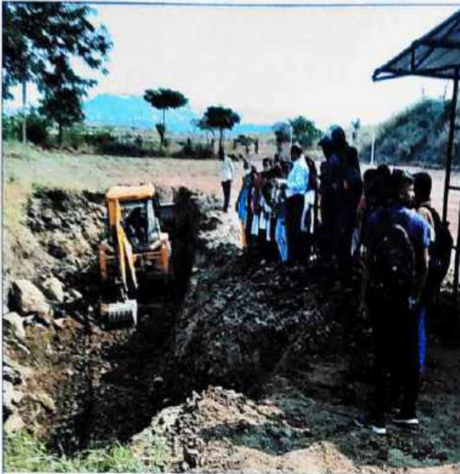
Principal giving information to the students while preparing rainwater harvesting pit
