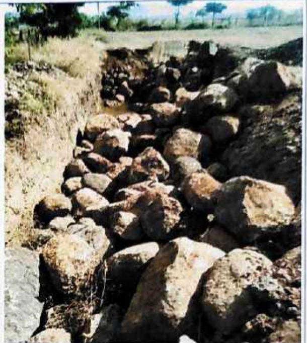
Pit filling with stone-brick
