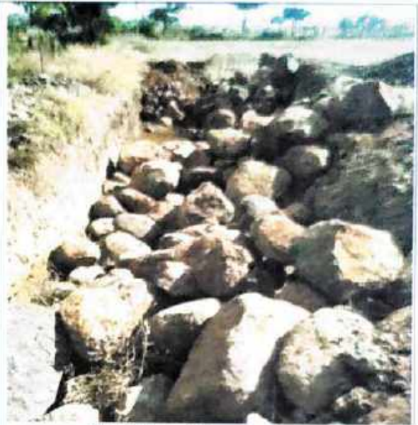
Pit filling with stone-brick
