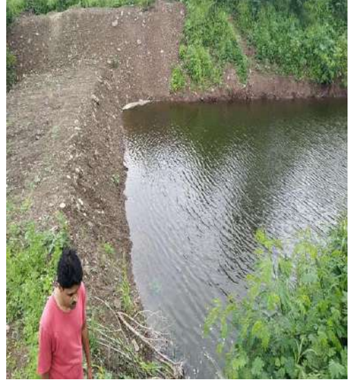
Water stored due to water conservation
