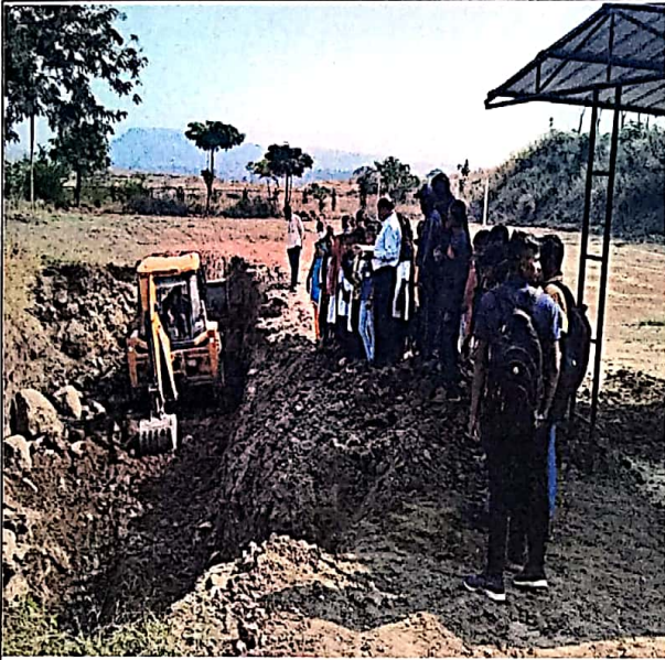
Principal giving information to the students while preparing rainwater harvesting pit
