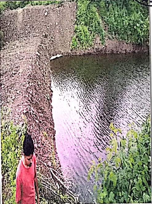
Water stored due to water conservation
