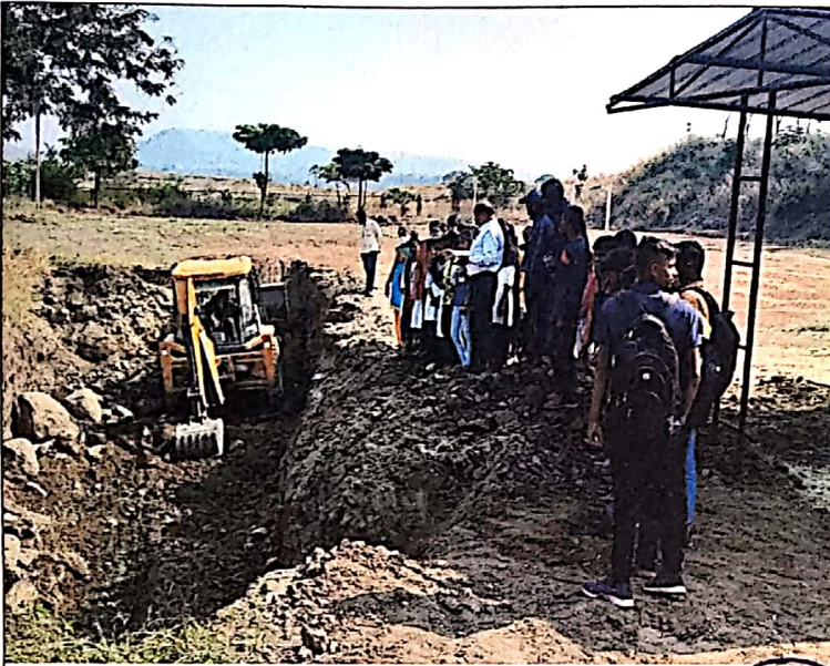
Principal giving information to the students while preparing rainwater harvesting pit
